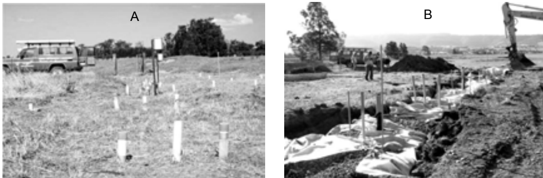
Figure 6. (A) Pilot-scale PRB with piezometers and monitoring wells in ASS terrain on Shoalhaven Floodplain, southeast NSW and (B) installation of the PRB
