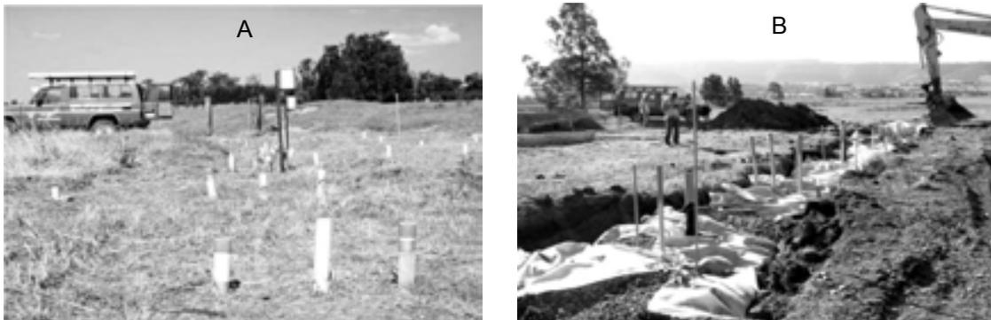
Figure 6. (A) Pilot-scale PRB with piezometers and monitoring wells in ASS terrain on Shoalhaven Floodplain, southeast NSW and (B) installation of the PRB
