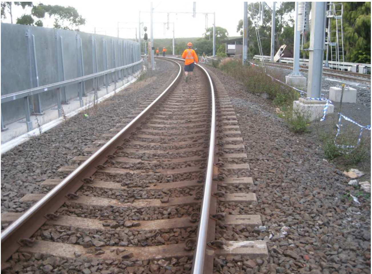
Figure 1 Typical ballasted railway tracks
