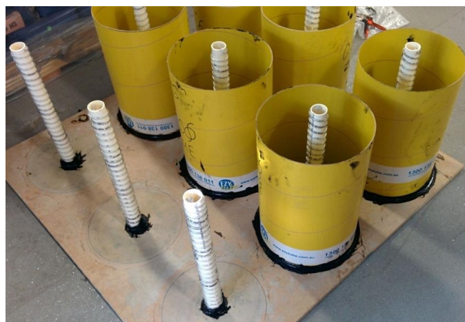
Figure 4: Completed moulds ready for casting
