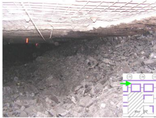
Figure 2: Crandall Canyon Pillar Burst Disaster (MSHA 2007)
