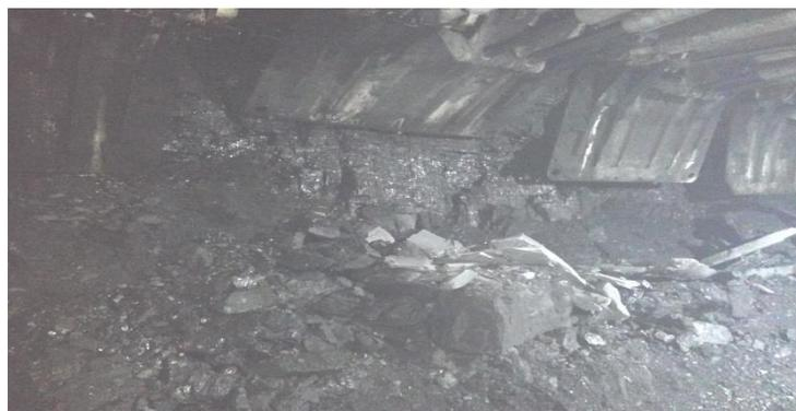
Figure 3: Rib spalling of LW12301 during first weighting
