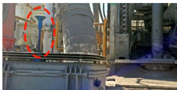
Figure 3: Dust monitor in use during drilling operations
