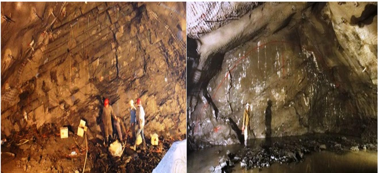
**Figure 4: Charging process and resulted profile after blasting**
