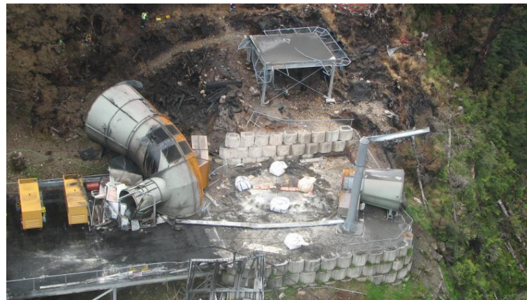
Figure 4 - The capped fan shaft, showing the evasee where it was deposited after the fourth explosion (NZ Police, 2012)
