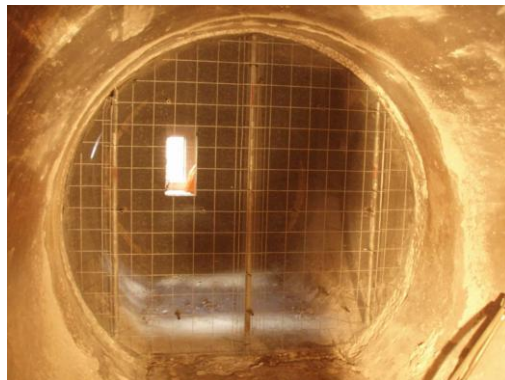
Figure 4 - Formwork for 100 mm seal
