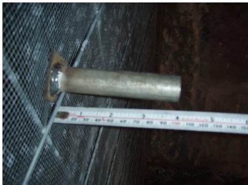
Figure 3 - Depth indicator attached to Tecmesh sheet formwork
