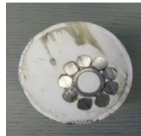
Figure 4 - Cross-section of 8 m Megadowel cables
