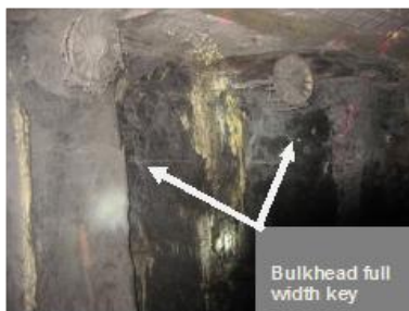
Figure 6 - Bulkhead 300 mm depth key with Tensar mesh removed and PUR injection of a central ring of holes
