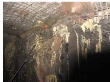
Figure 7- PUR injection of upper rib Mudstone interbedded with coal lenses
