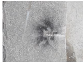
Figure 15 - Split surface of the blasted area
