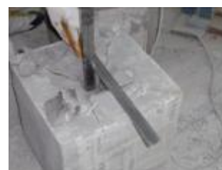
Figure 6 – Measuring the cavity depth
