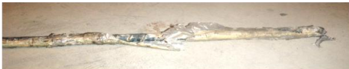
Figure 2 - Overcored bolt taken from the support pattern
