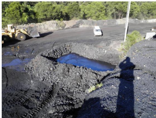
Figure 6 - Dam composed of loose rocks
