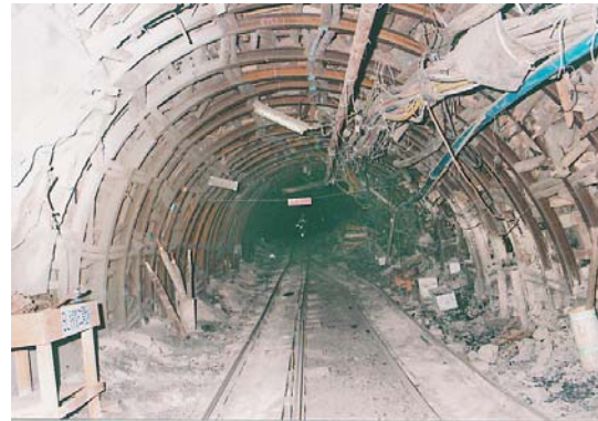
Figure 9 - Side tunnel, near Node 3B
