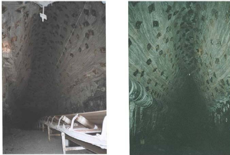
Figure 4 - Standard “Failure Arch” roadway roof fall cavities at Crinum Mine (Payne 2008)
