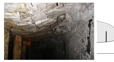
Figure 14 - Common roof deformation pattern is consistent with outer bolts being the only ones anchored
