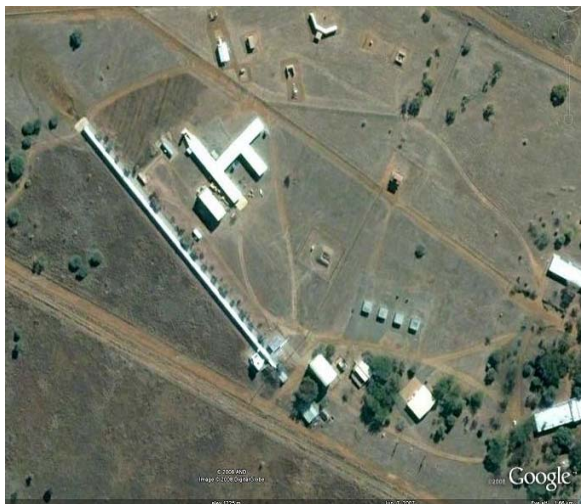
(a) Aerial view
