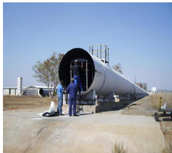
(b) At the mouth of the tunnel
