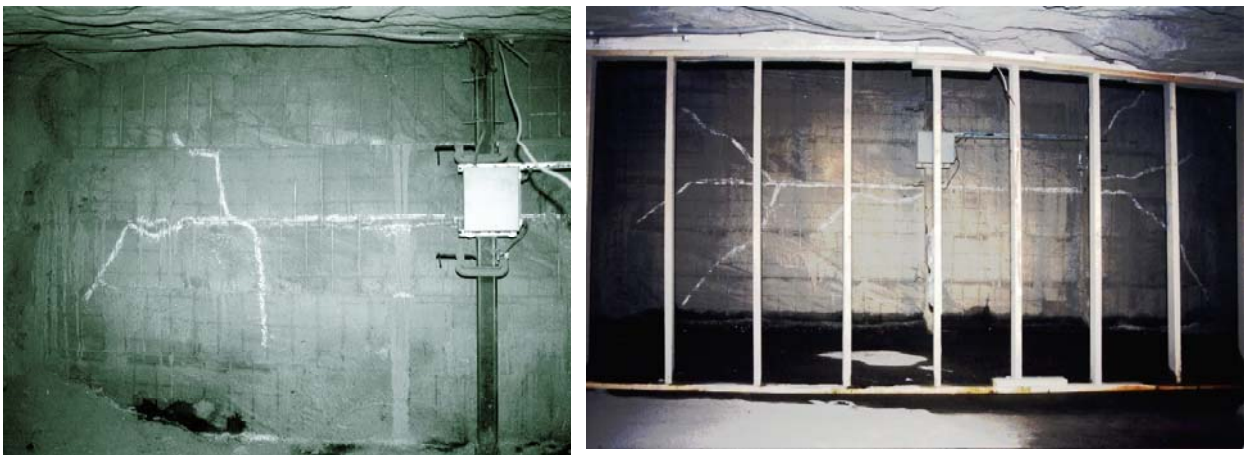
Figure 3 - Formation of yield lines in Meshblock™ seals
