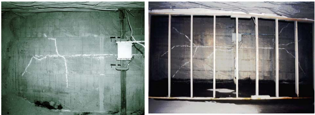
Figure 3 - Formation of yield lines in Meshblock™ seals
