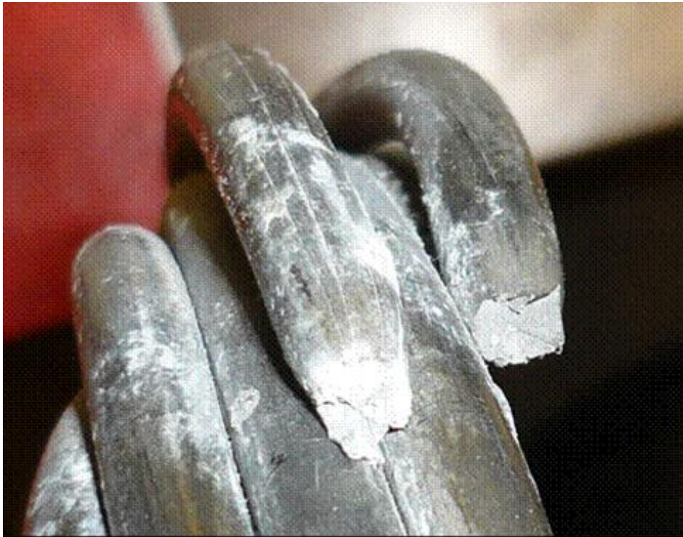
Figure 9 - Cone and Cup strand failure
