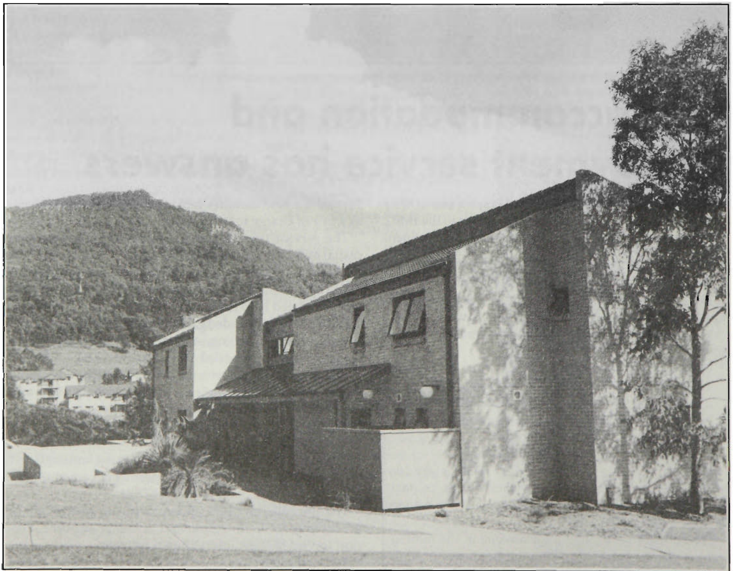
University Lodge. The front entrance off Northfields Ave. Kooloobong is in the background
