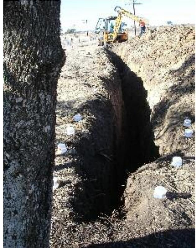
Figure 38 Trench excavation to examine the root density distribution of a native tree (Miram, VIC, Australia)
