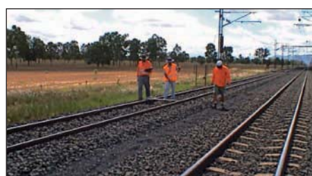
Figure 1: Corrugation tests in a typical ballasted railway track in Central QLD.
