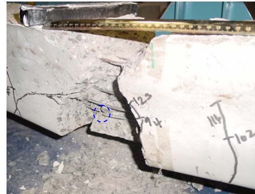
Figure 10: Prestressing wire damages
