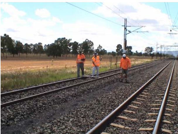
Figure 1. Typical ballasted railway track in Australia
