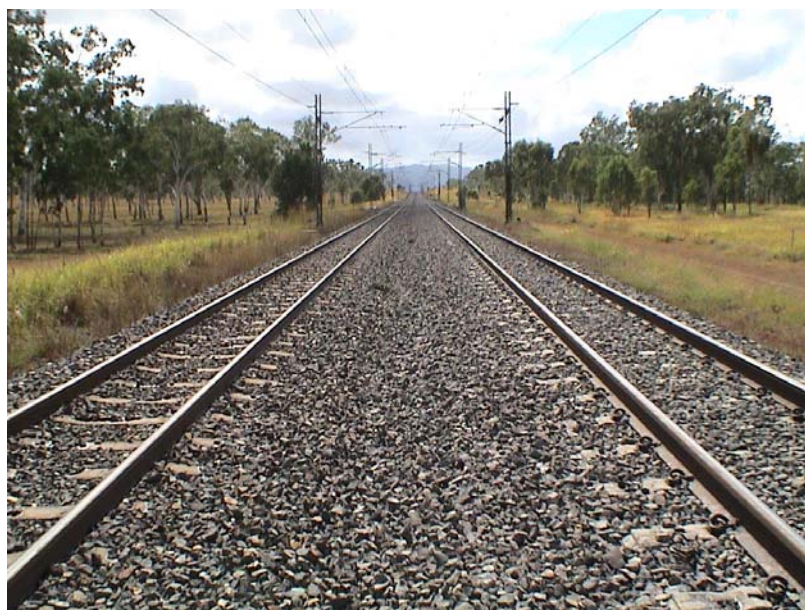
Figure 1: Typical ballasted track on a coal line in Central Queensland (after [7])
