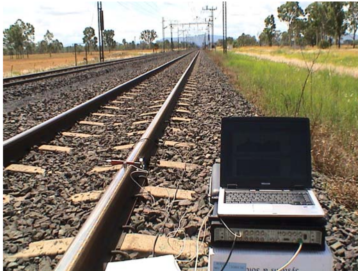
Figure 4: Dynamic testing installation
