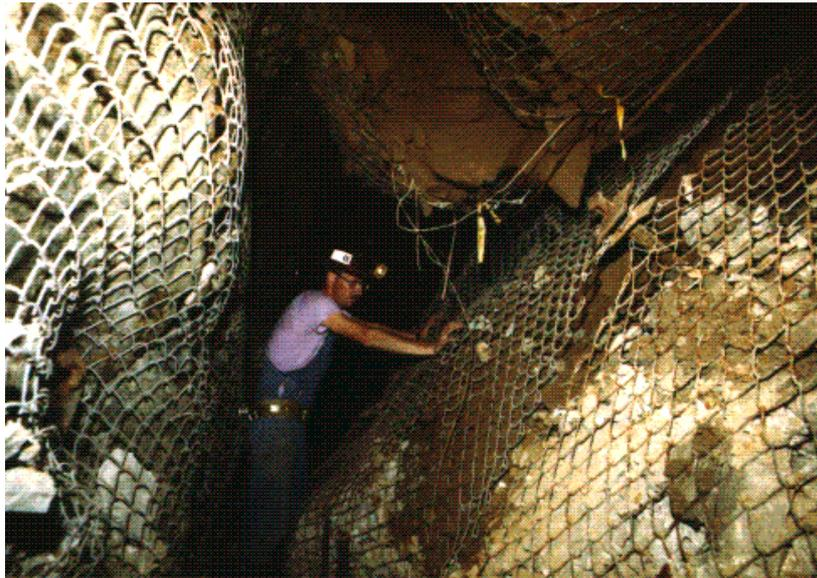
**Fig. 1 Damage to a drive from rockburst**
