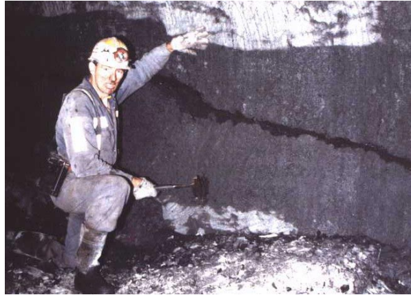
Plate 1. A normal fault in the Bulli seam – Southern Coalfield - normally 2-3m thick. The effect of the fault has been to reduce the mining height to about 1m. The trace of the fault plane can be seen as the heavy black line (centre) with sandstone in both the roof and floor.
