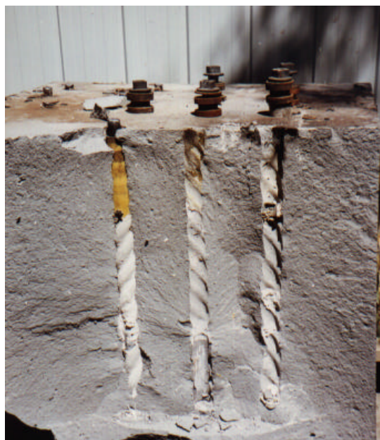
Fig 2 - Rifled drill hole
