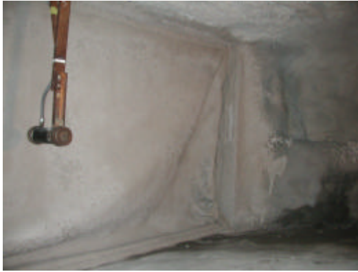
Fig 14 – Finished stopping cut-through 6
