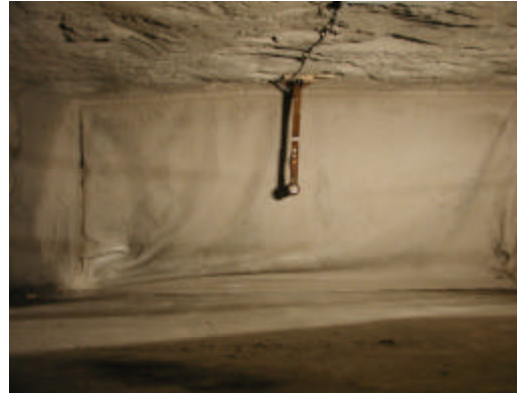
Fig 15 – Finished stopping cut-through 7
