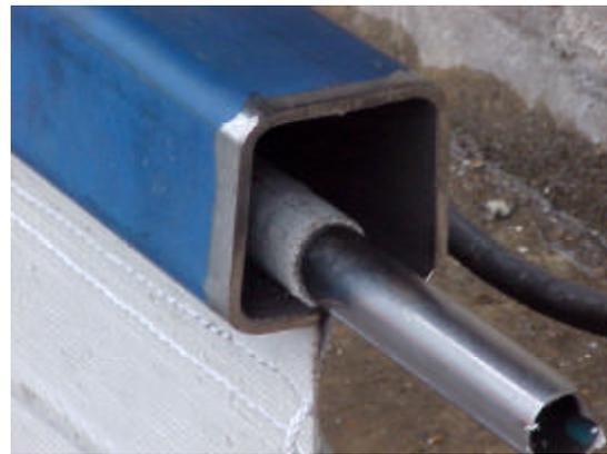
**Fig 7 - Slot fixing system**
