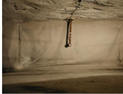
**Fig 15 – Finished stopping cut-through 7**
