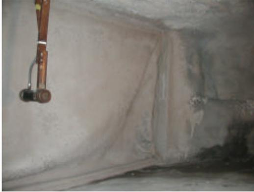
**Fig 14 – Finished stopping cut-through 6**
