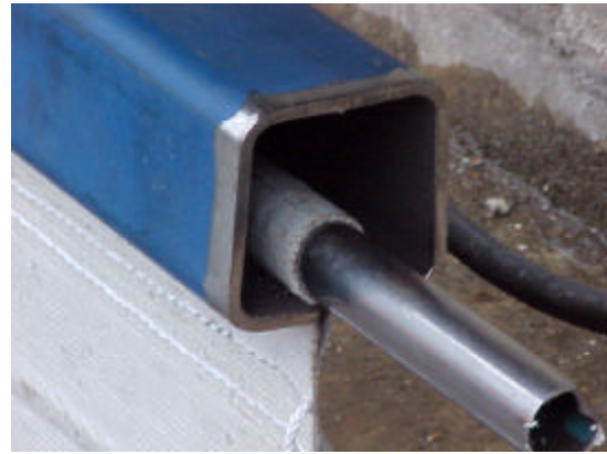
Fig 7 - Slot fixing system
