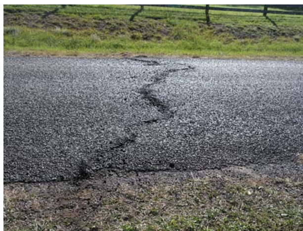
Figure 3 - Mining-induced surface wrinkles
