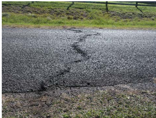
Figure 3 - Mining-induced surface wrinkles
