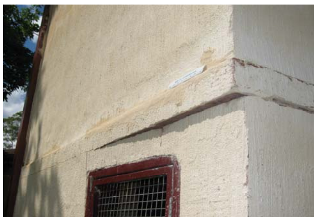
Figure 1 - Structures Affected by Horizontal Shear Deformations
