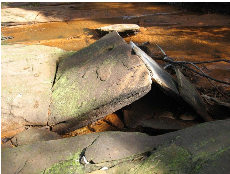
Figure 2 - Buckling of near-surface, Waratah Rivulet, late 2004
