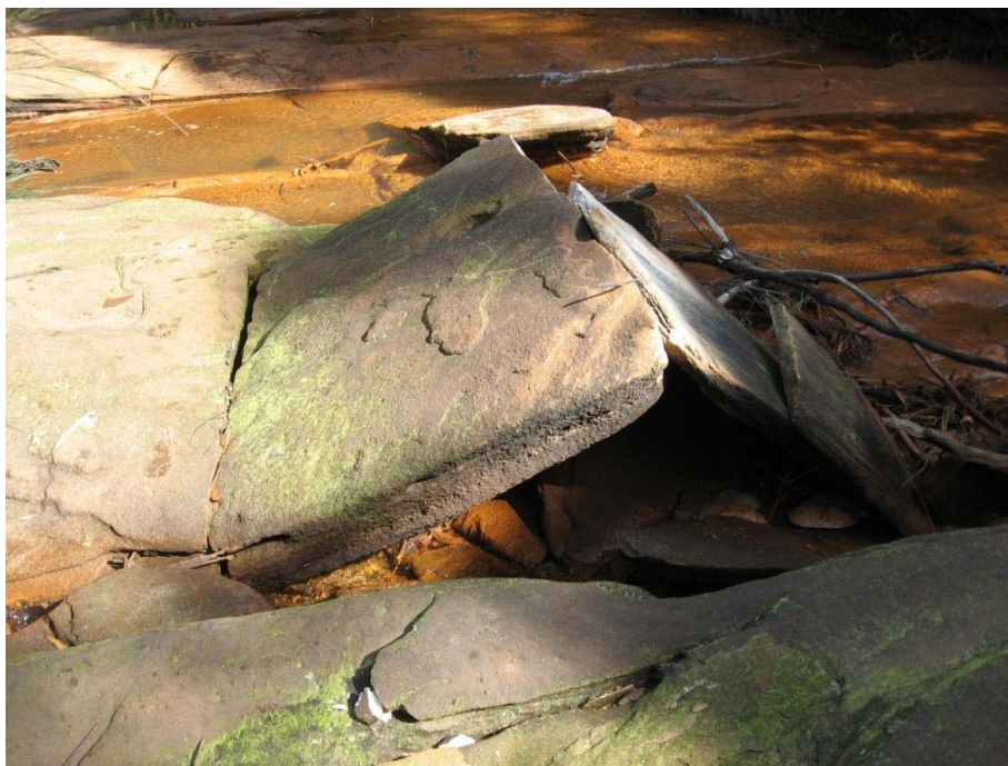
Figure 2 - Buckling of near-surface, Waratah Rivulet, late 2004
