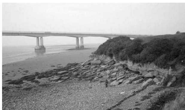
Figure 14. Boulder accumulation fanning upstream in the Severn Estuary (toward viewer) along cliffs at Sudbrook, South Wales (standing figure for scale).
