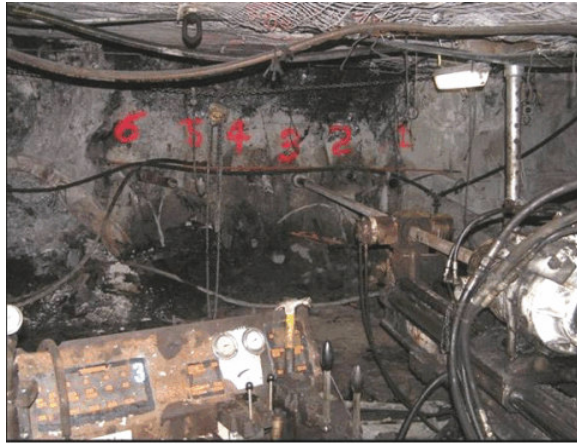
Fig 3: Photograph of Douglas pit bottom site showing the location of the six 50m long boreholes used for the casing trial.
